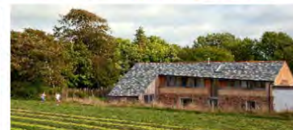
Above: The Cob has been converted into holiday accommodation from a former agricultural building.
